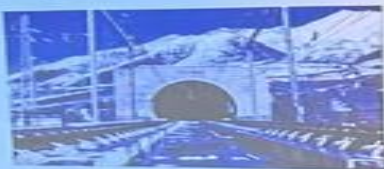
Railway Tunnels in Plateau Areas
