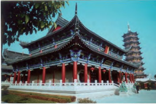
The columns in oriental building
