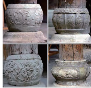
The pedestals of columns
