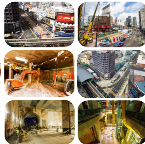
Excavation stages for the underground construction
