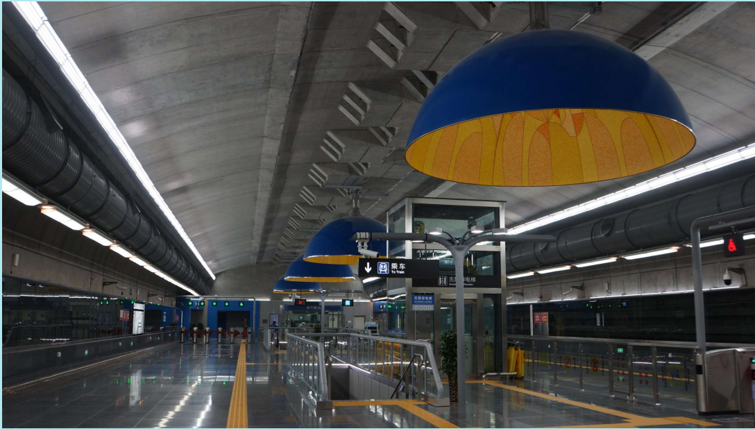
Shuangfeng Station of Changchun Metro Line 2 in operation
